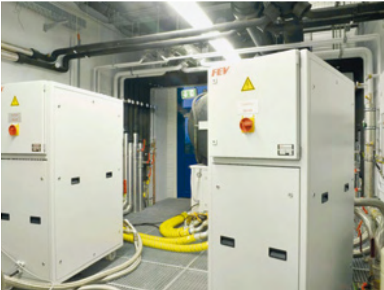
Figure 4: Multi functional technical area between each two test cells – here shown with mobile systems for coolant conditioning and thermo shock
