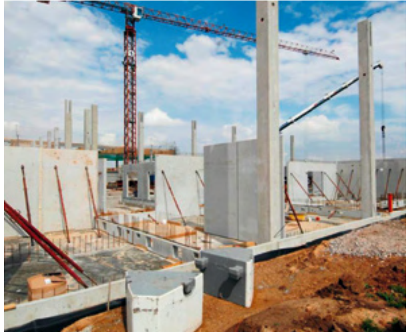
Figure 7: Test cell construction with concrete modules
