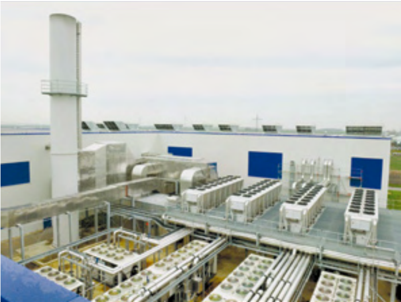
Figure 10: Generation of cold and cooling water at the central technical area
