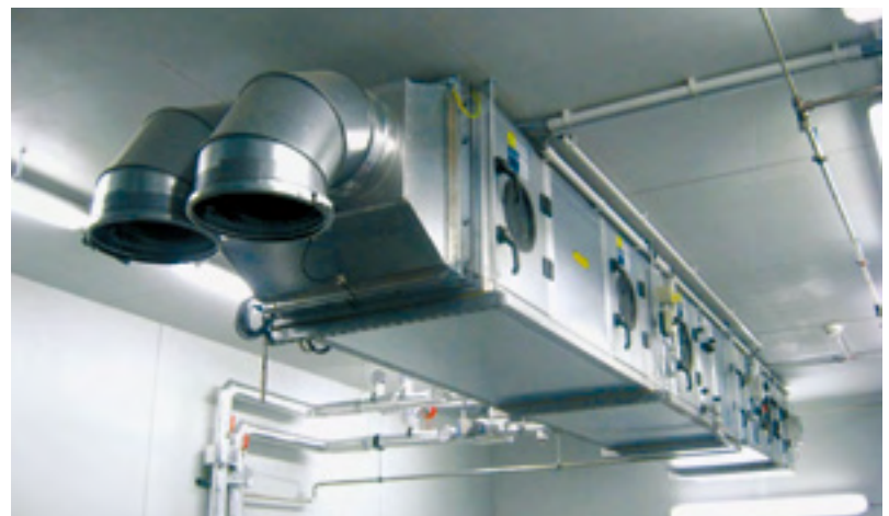
Figure 15: Venting device in TC for standard combustion air tempering
